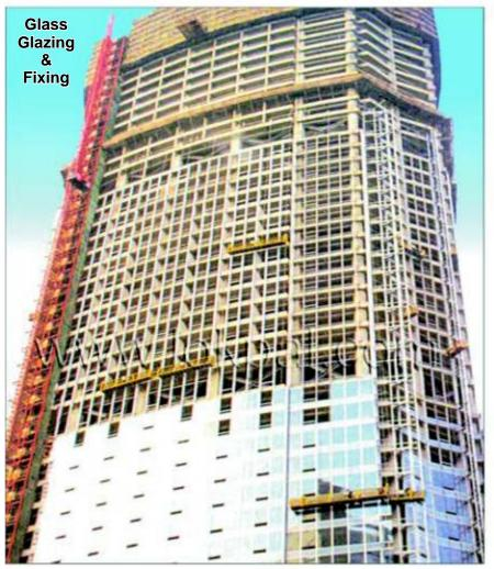
A large number of commercial high-rise buildings in India now have external glass curtain walls. Such buildings require constant maintenance, This is highly dangerous work which should be carried out by cleaners using Suspended Cradle System with a Cradle suspended from the roof which replaces conventional scaffoldings. The system can be used for external brickwork, plastering, painting, finishing etc.
