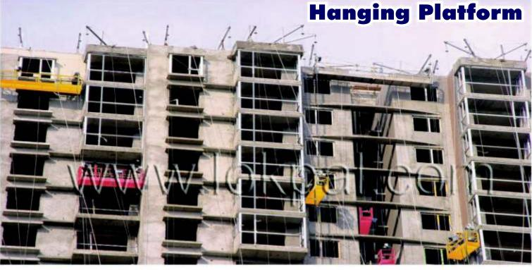
Cradle Systems being used for Finishing, Plastering, Painting, Glass Fixing and Aluminum Fixing
